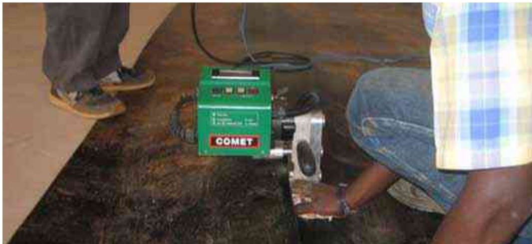
Figure 4.17: Proof of welding seams 21
