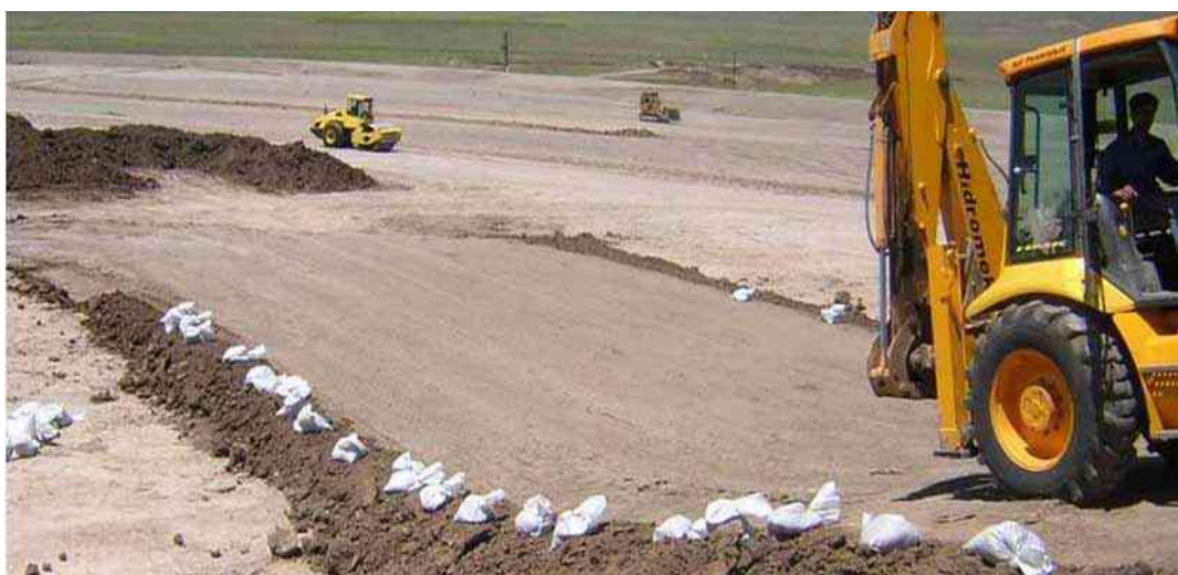
Figure 4.14: Construction of Test Field 18
