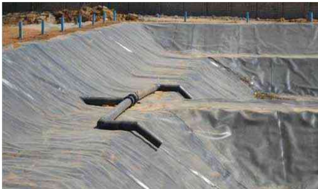
Figure 4.10: Sealed Leachate Pond with Two Basins 14
