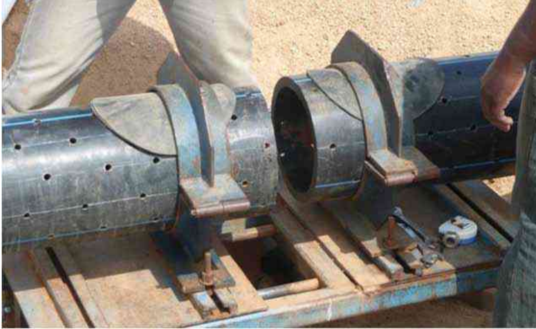
Figure 4.19: Proper Holed Leachate Pipes 24
