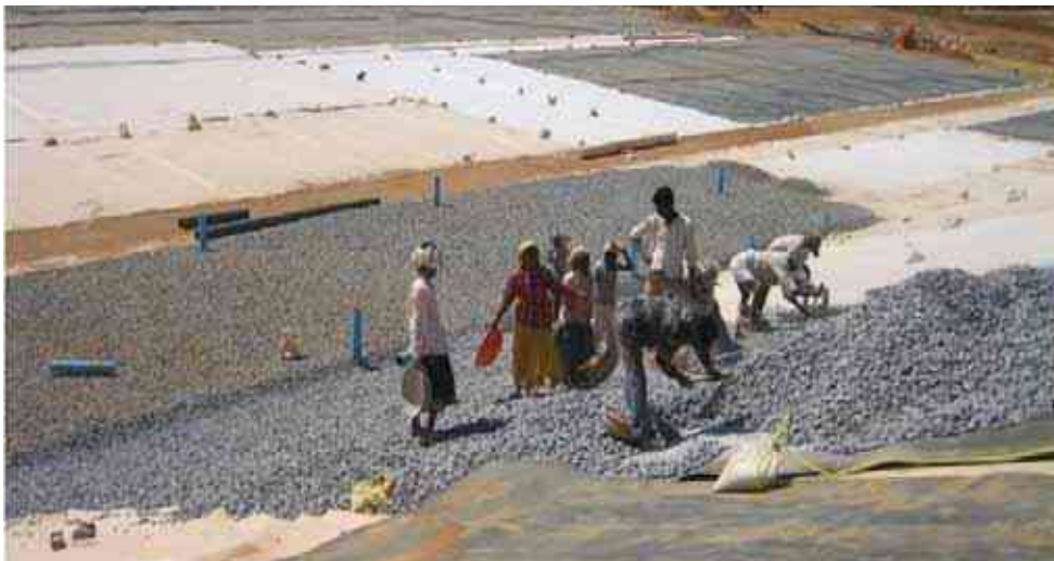
Figure 4.13: Sanitary Landfill under Construction 17
