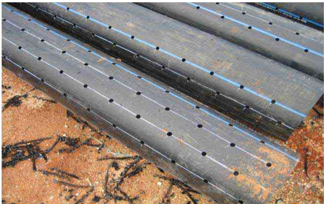
Figure 4.18: Welding of Leachate Pipes 23
