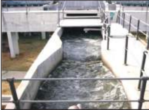
Figure 5.34 Typical Parshall Flume Installation
