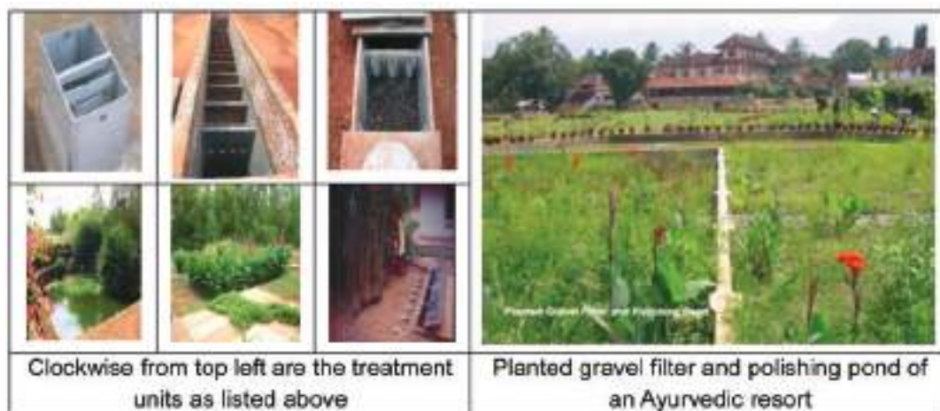
Figure 8.15 Typical DEWATS treatment plant components
