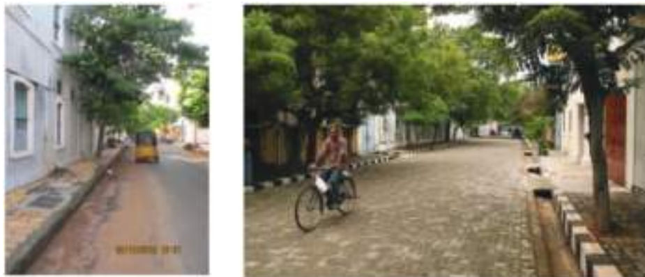
Figure 8.6 Simplified sewerage in the footpath and main road free of manholes in French Puducherry - early 20 th century
