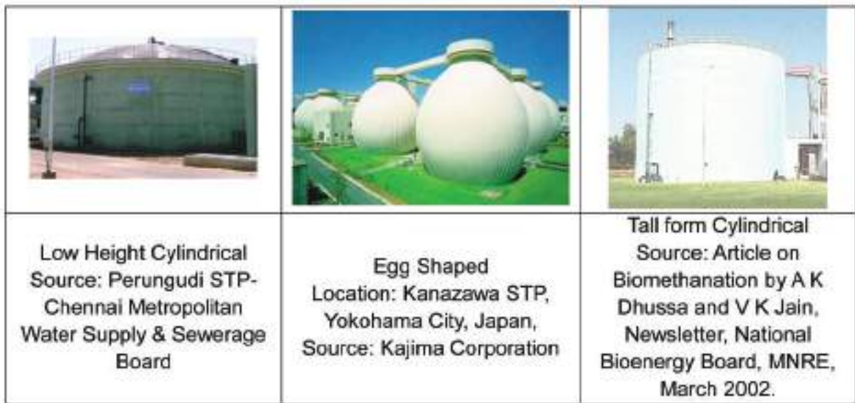
Figure 6.8 Typical low height cylindrical, egg shaped and tall form cylindrical digesters
