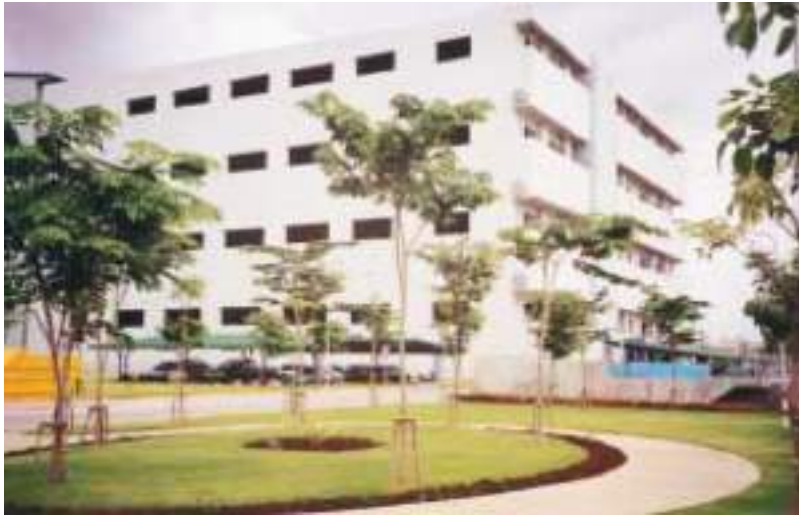
Figure 5.81 Yannawa STP, Thailand
