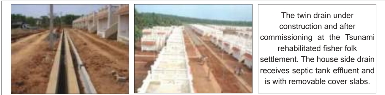
Figure 3.11 Twin drain system
