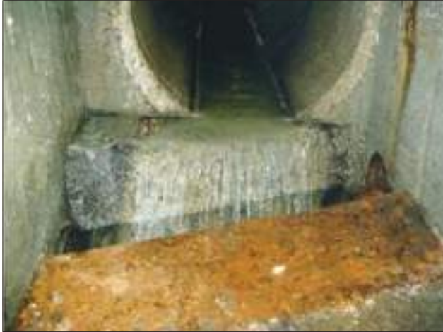
Figure 3.17 Typical floor level leaping weir
