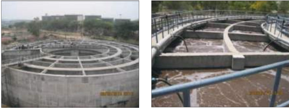
Figure 5.16 Left is the bioreactor during construction; Right is the bioreactor after commissioning showing the rich MLSS culture in the annular plug flow reactor
