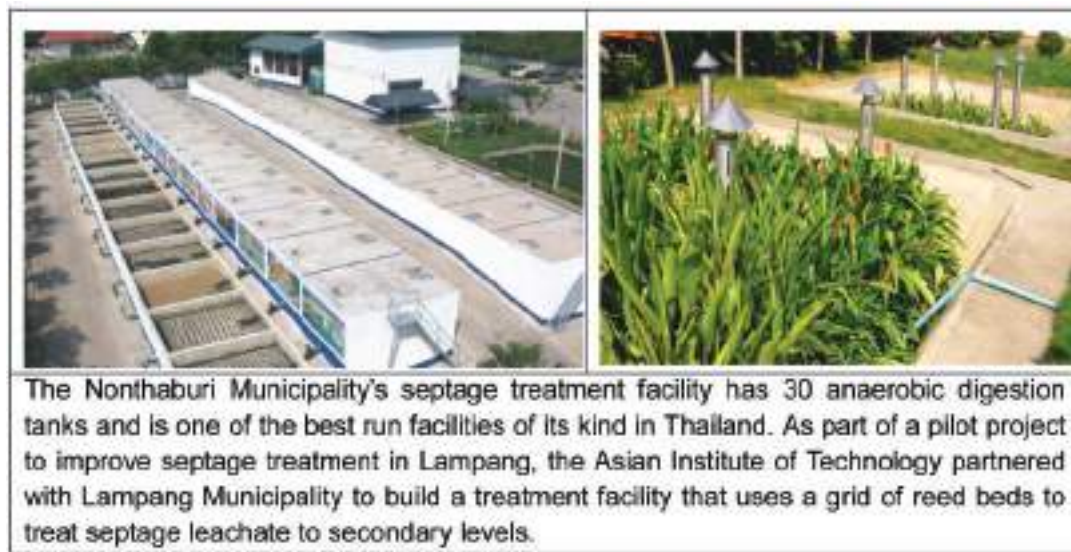
Figure 9.21 A photo view of seepage treatment process at Nonthaburi in Thailand
