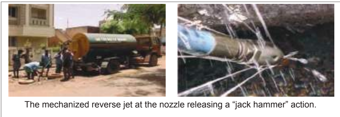
Figure 3.10 Jet rodding cum vacuum, suction sewer cleaning machine
