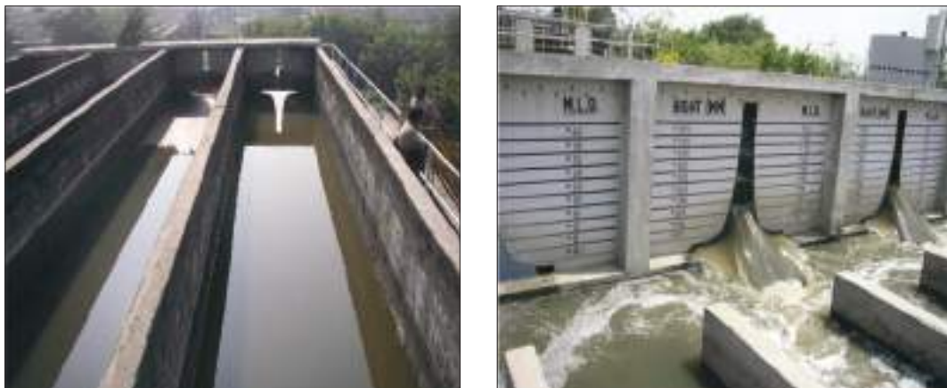
Figure 5.31 Typical Installation of proportional flow weir.
