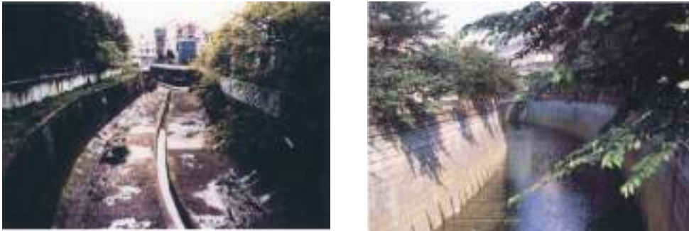
Figure 7.17 Condition of Meguro River (a) before and (b) after the restoration using reclaimed wastewater
