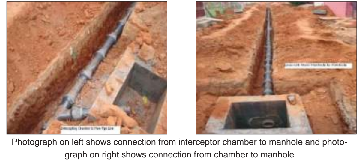
Figure 3.18 House sewer connections
