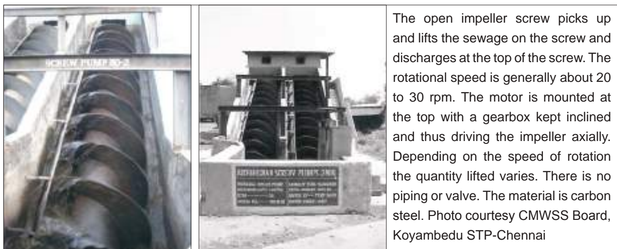
Figure 4.4 Archimedeian screw pump.
