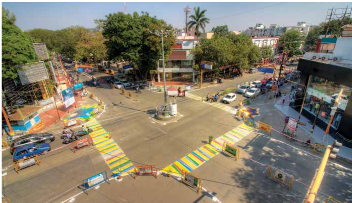
Fig. 27 Testing of a Proposed Intersection Design in Coimbatore
