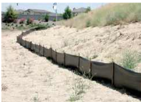
Figure 6. 6: Silt Fence
