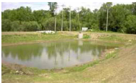
Figure 6. 4: Sediment Basin
