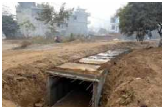
Figure 11. 7: Box drain
