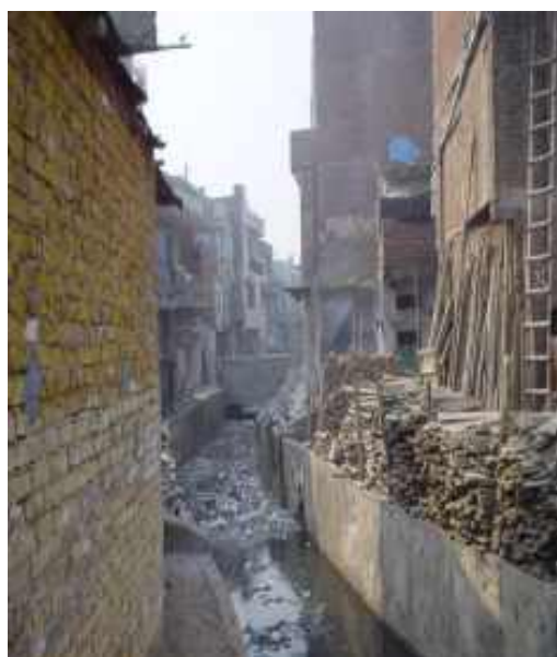
Figure 1.4: Encroachment in storm water drains
