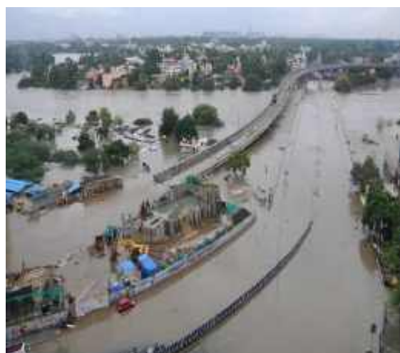
Figure 1.1: Adyar River flowing over the Saidapet Bridge in Chennai flood in 2015
