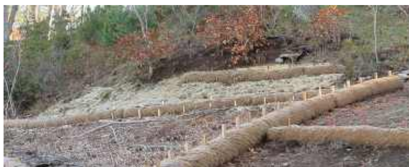
Figure 6.7: Brush Barrier
