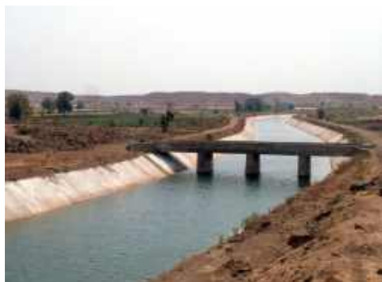
Figure 5. 14: Concrete Channel
