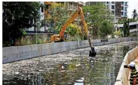
Figure 2. 2: Cleaning of drains in Mumbai
