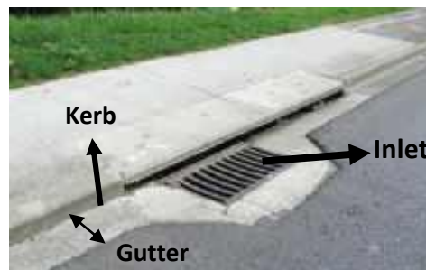
Figure 5. 4: Gutter and Inlet
