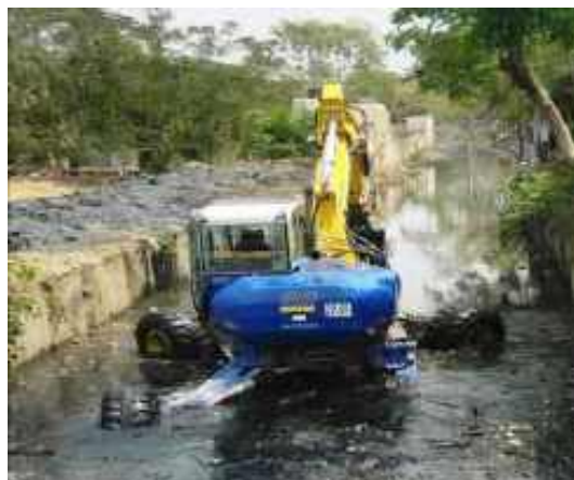
Figure 2. 3: Robotic Excavator in Chennai
