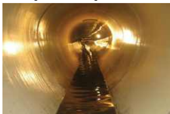
Figure 1.3: Rehabilitation of Brick Combined Sewer in Kolkata
